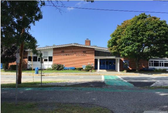
H1. Hatherly Elementary School main entrance.
