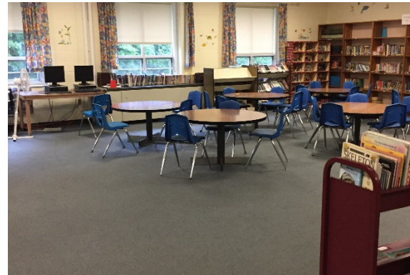
W11. Carpeting in the library smells of mildew, is worn, and should be replaced.
