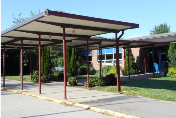
W1. Wampatuck Elementary School main entrance.
