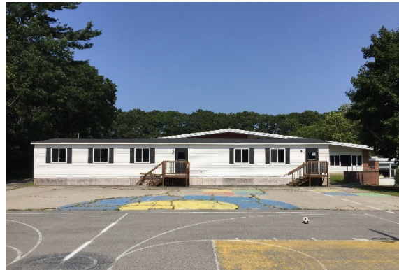
C5. The modular building has exceeded its useful life. Entrances are not code compliant.
