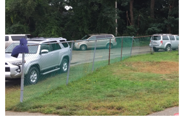
W3. Chain link fences are badly rusted and damaged throughout the site.
