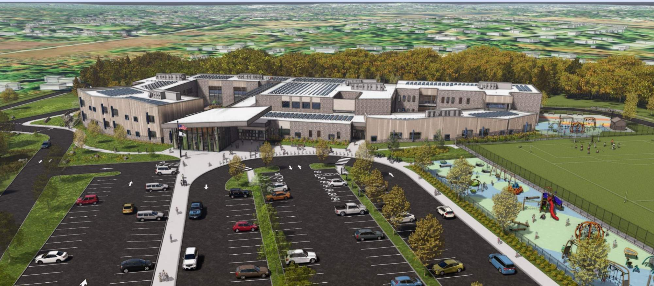
Aerial View Looking West
