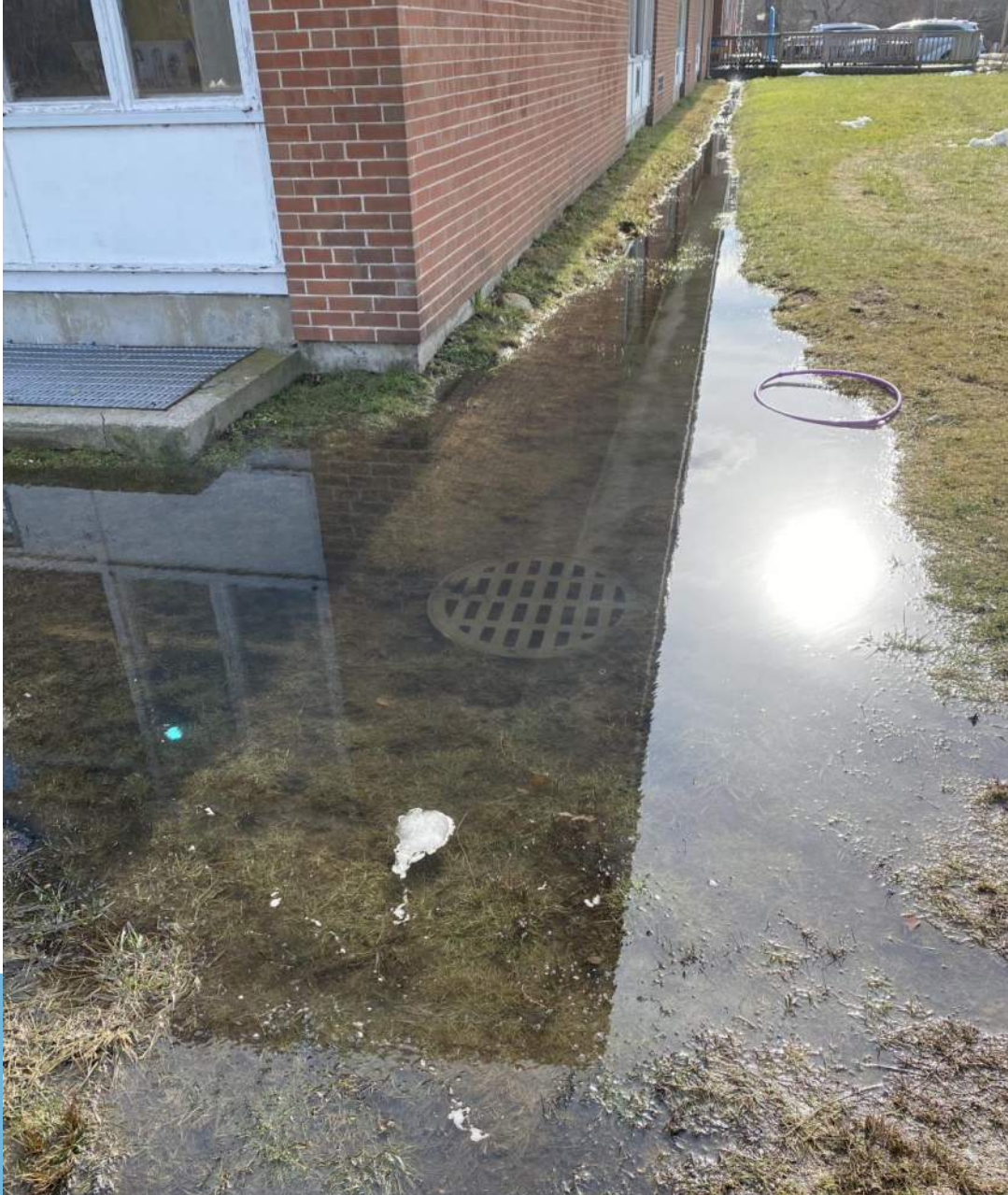
Clogged site drains, poor soil drainage
