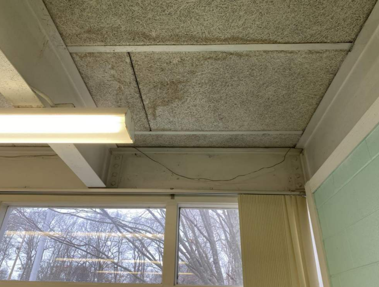
Roof leaks, roof decking not easily repairable
