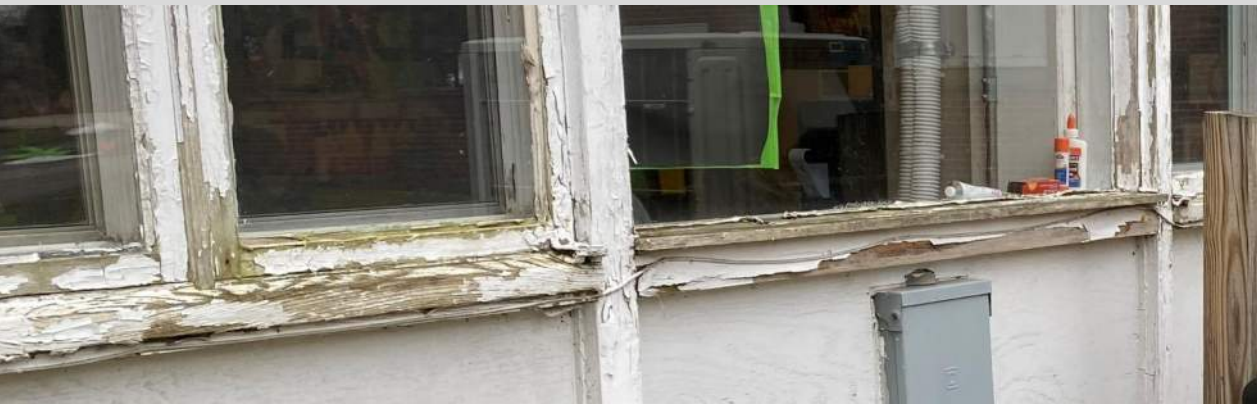
Peeling, rotted wood windows, poor insulation
