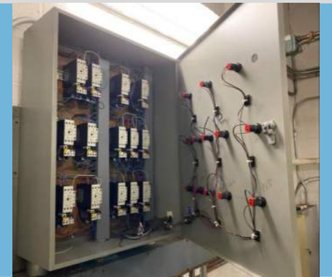
Original 1960's Electrical Switchgear, Controls
