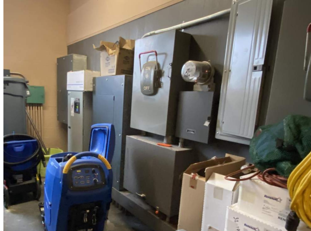
Original 1960's Electrical Switchgear, Controls
