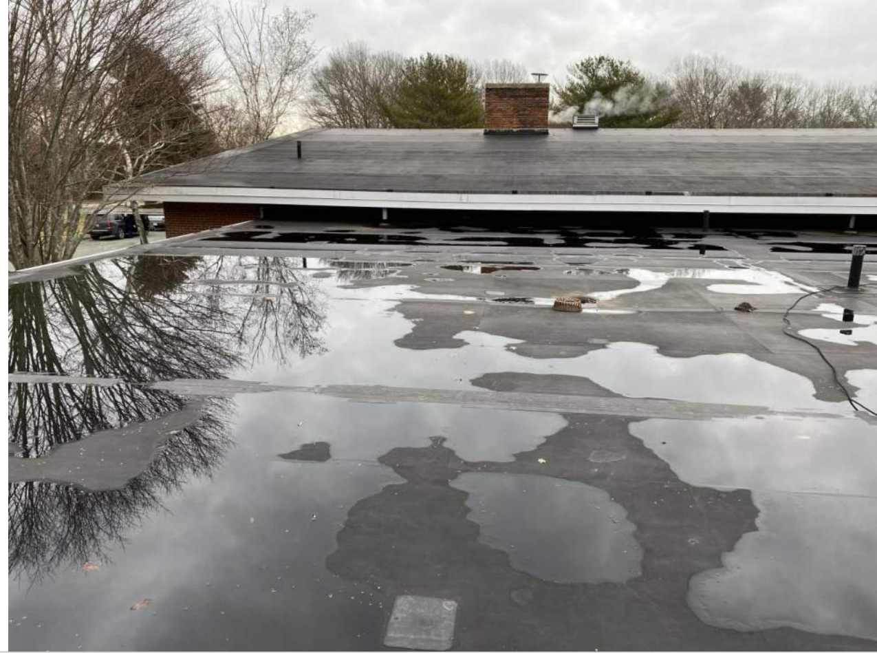
Inadequate roof pitch, leaks
