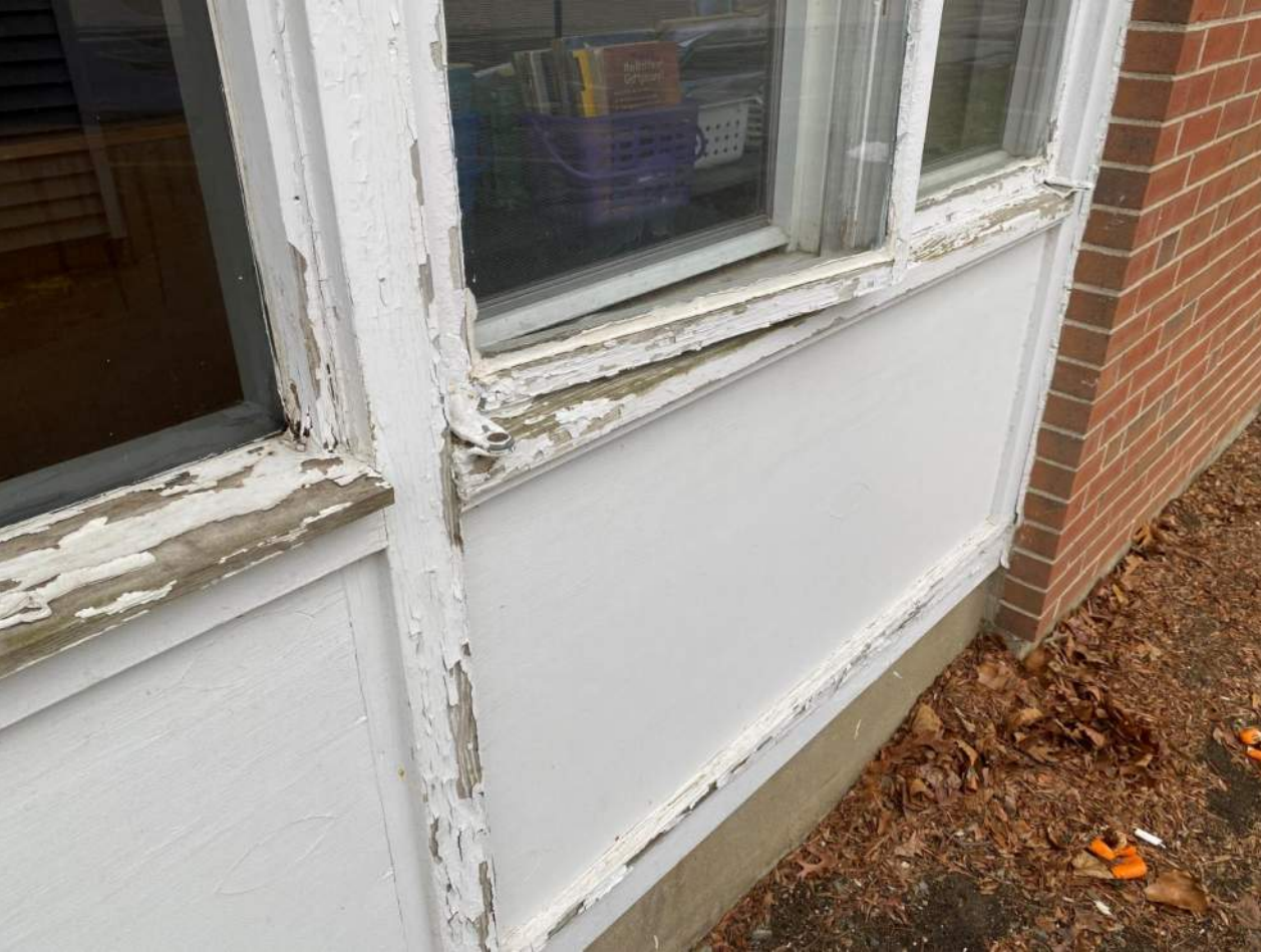
Peeling, rotted wood windows, poor insulation
