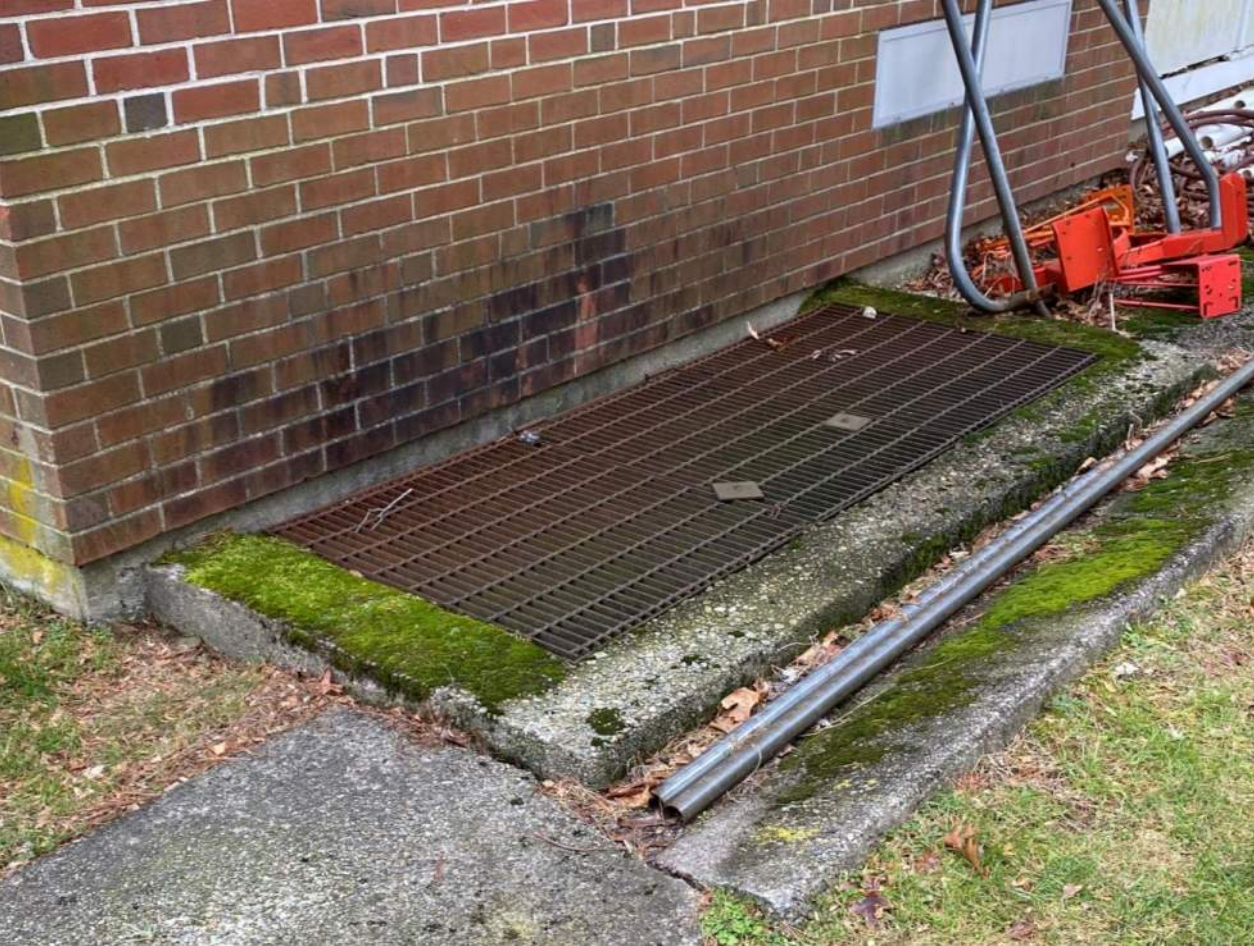
Moisture issues at brick, poor insulation
