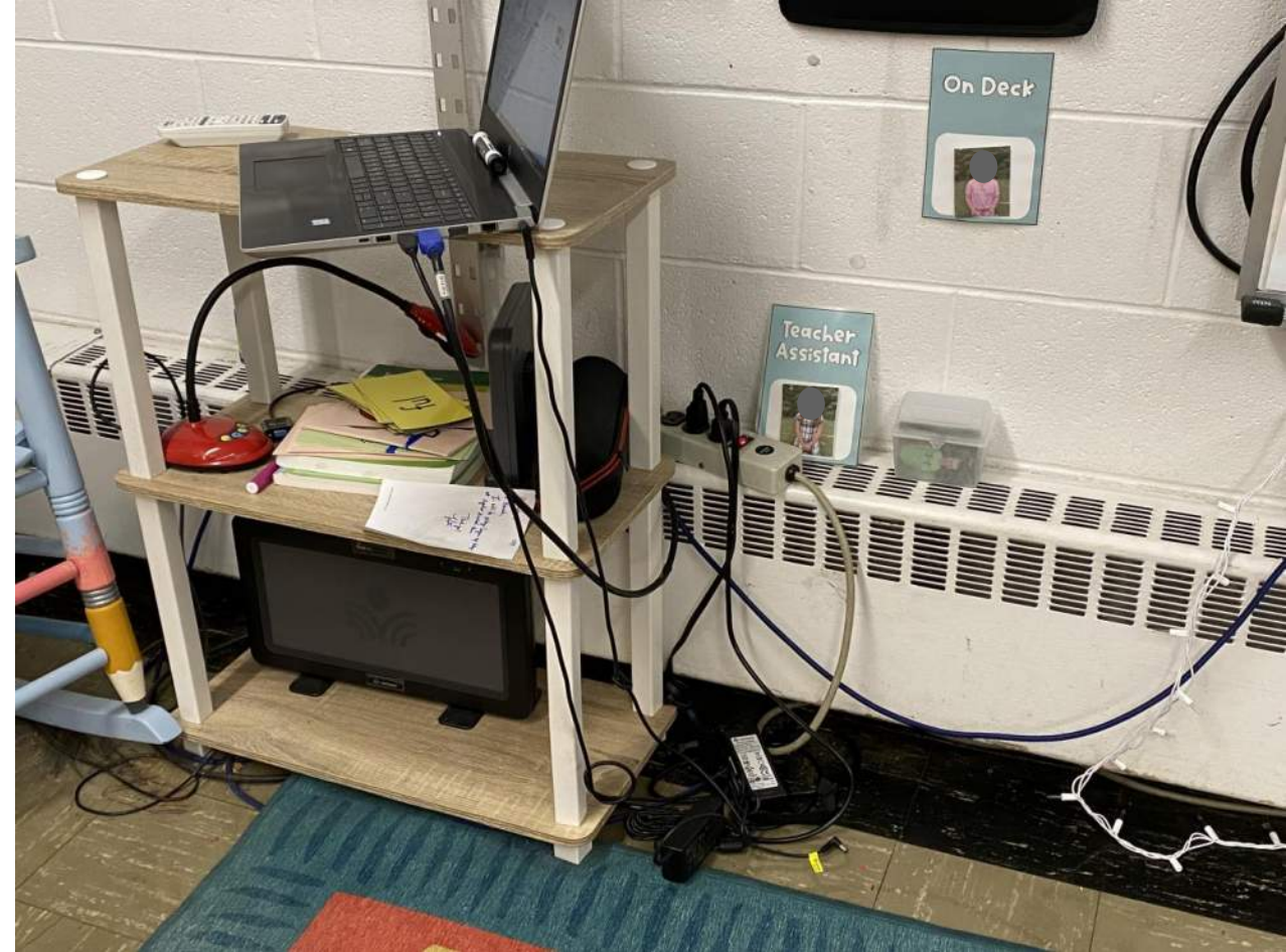
Insufficient Electrical Outlets, power strips used
