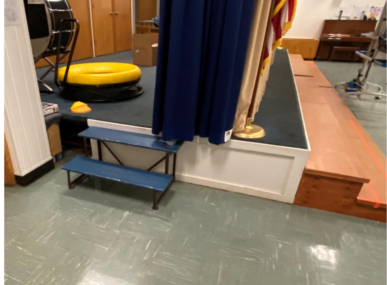
Non-accessible stage platform at Cafeteria
