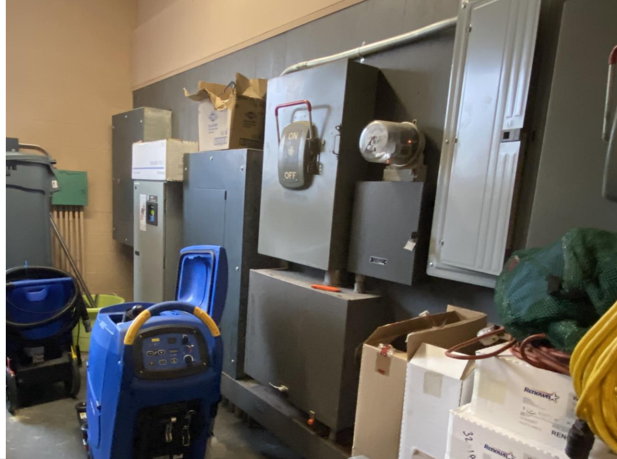
Original 1960's Electrical Switchgear, Controls
