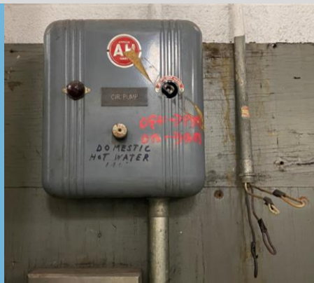
Original 1960's Electrical Switchgear, Controls
